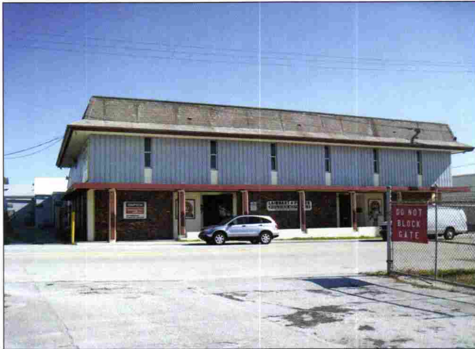
Photograph 1. View of main facade, facing northeast (PCI March 2010).
