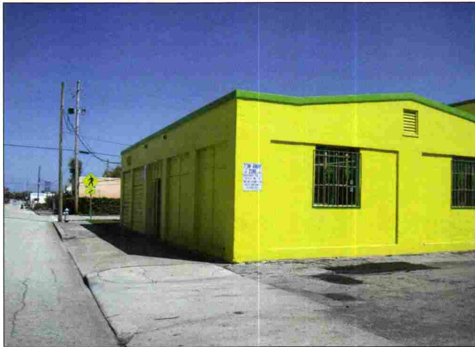
Photograph 2. Detail of office block, facing northeast (PCI March 2010).
