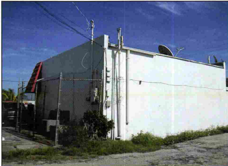
Photograph 2. Rear façade of PB14842, facing southeast (PCI March 2010).
