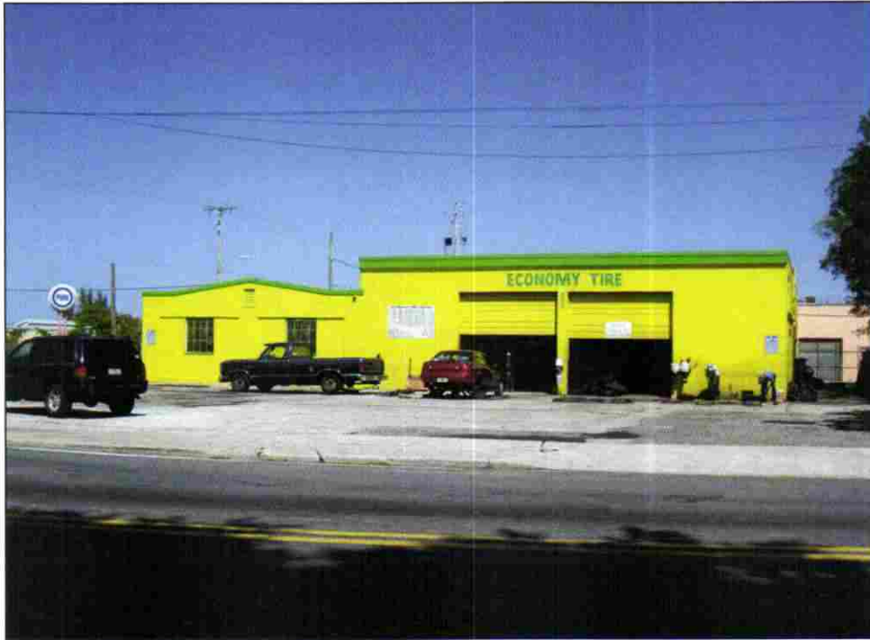
Photograph 1. View of main façade, facing east (PCI March 2010).
