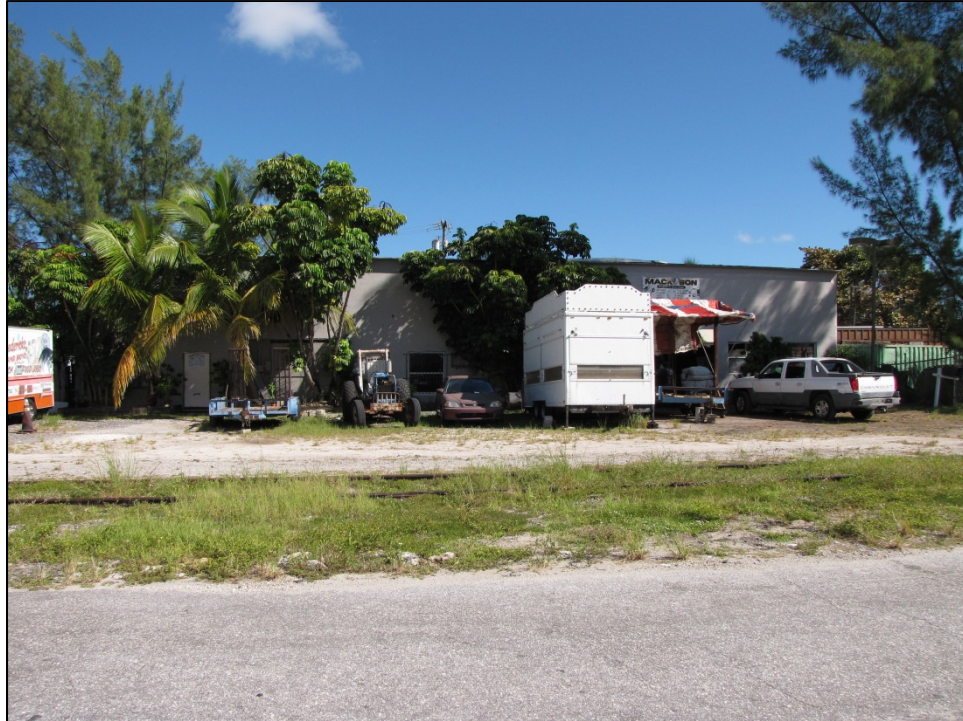
Figure 9: Mack and Sons (8PB16053), located at 921 27 th Street, facing North
