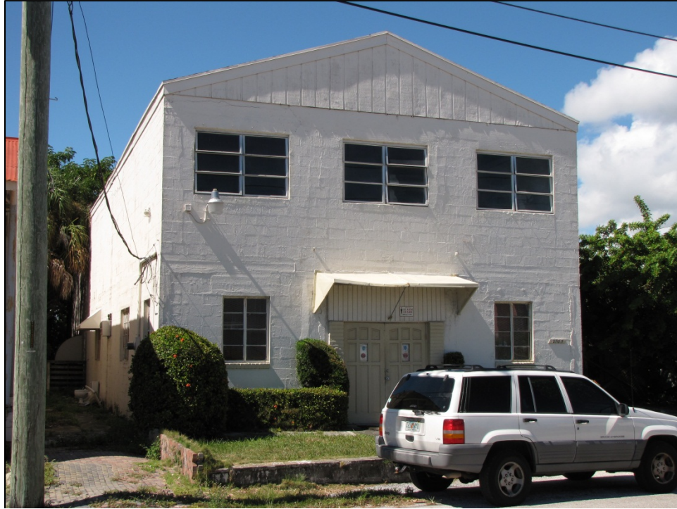
Figure 14: 2705 Division Avenue-Building #1 (8PB16058), facing Northwest
