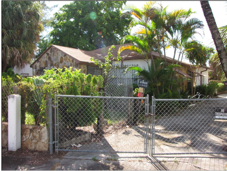
Figure 8: 974 29th Street (8PB16052), facing Southeast
