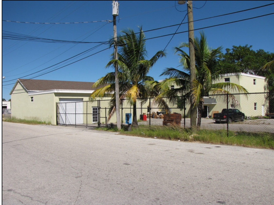
Figure 17: 2616 E. Tamarind Avenue (8PB16061) at 7525 NW 37 th Avenue, facing Northeast
