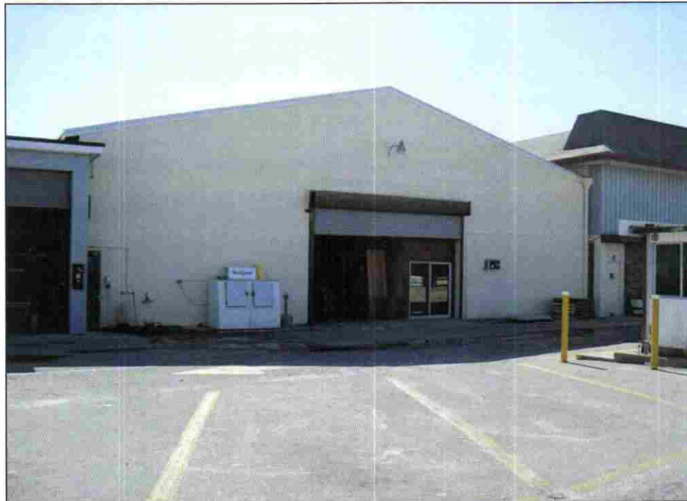
Photograph 2. View of rear facade, facing southeast (PCI March 2010).
