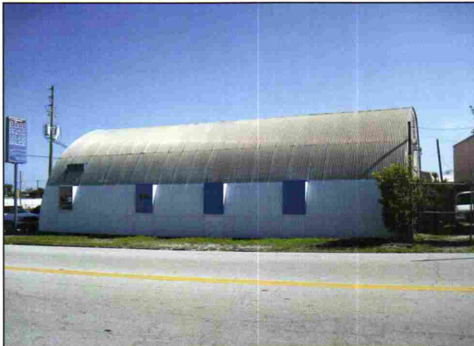
Photograph 2. View of north façade, facing southwest (PCI March 2010).
