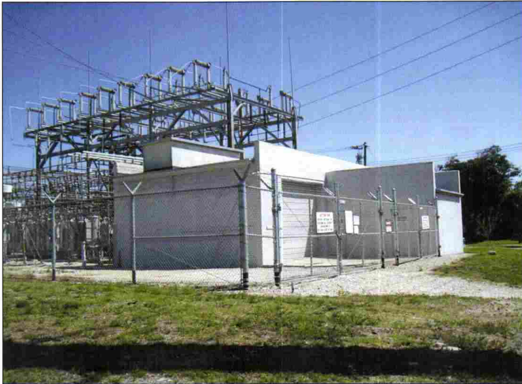
Photograph 1. View of substation, facing southeast (PCI March 2010).
