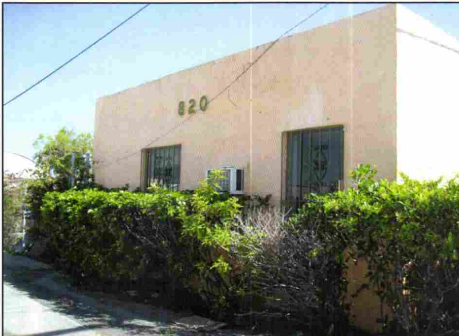
Photograph 2. View of north façade, facing southeast (PCI March 2010).
