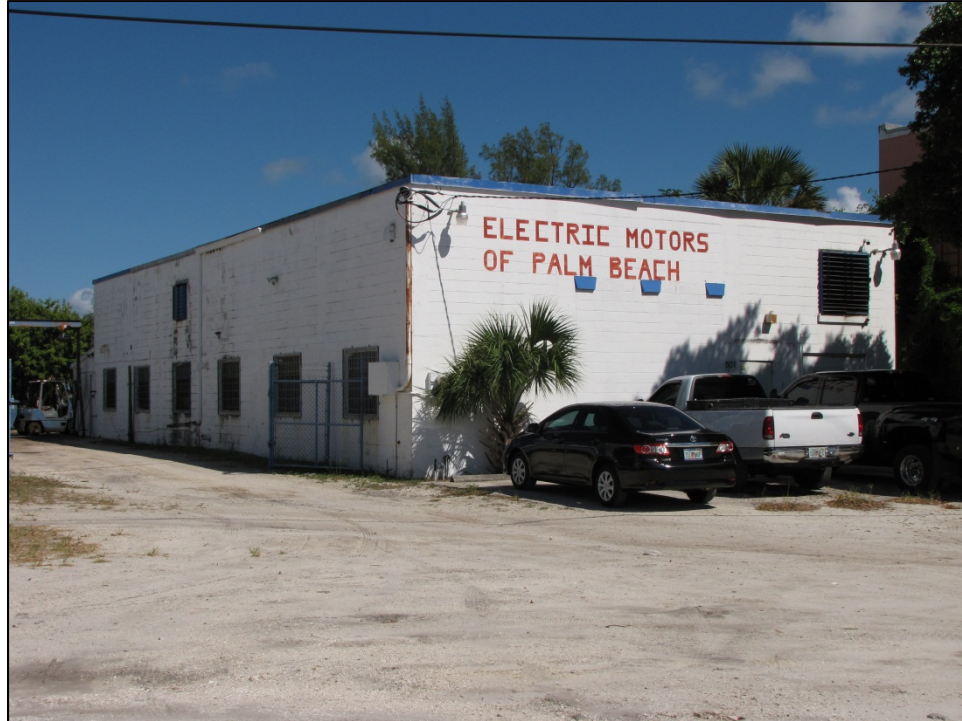
Figure 13: Electric Motors of Palm Beach (8PB16057), located at 801 27 th Street, facing Northeast
