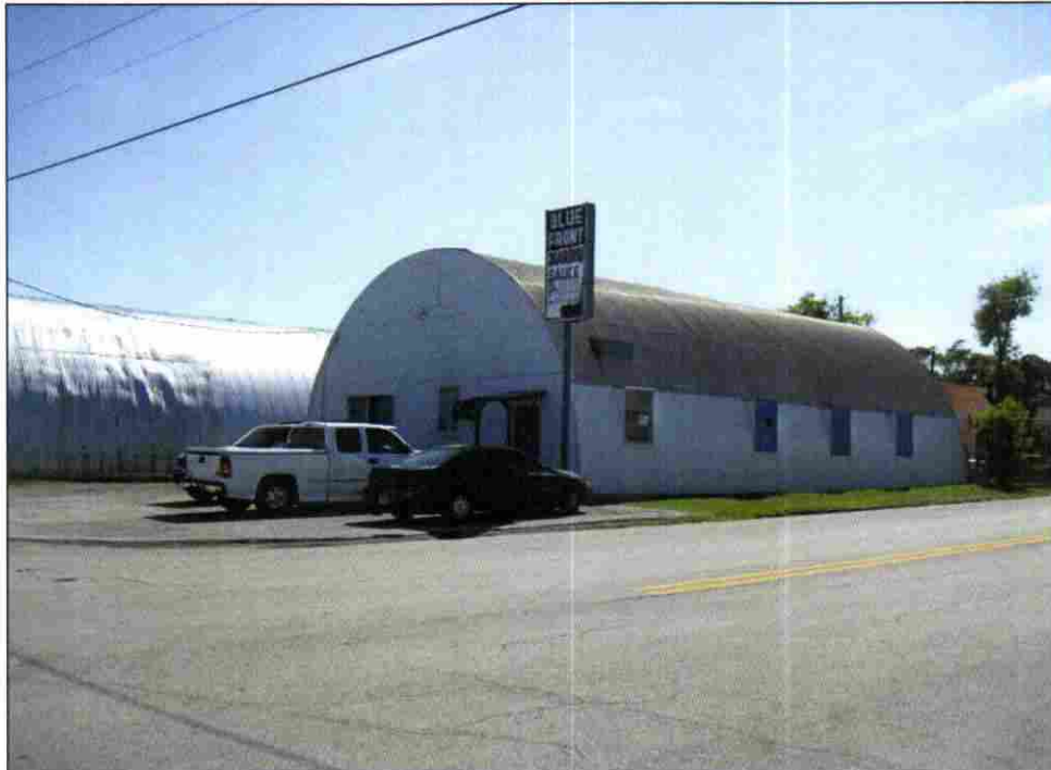
Photograph 1. View of main façade, facing southwest (PCI March 2010).
