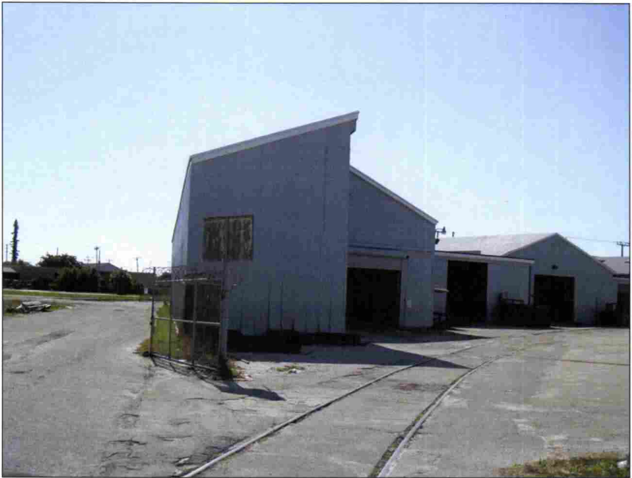
Photograph 1. FEC-SAL Railway Connector, facing east (PCI March 2010).
